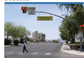
Pedestrian Flashing Beacons
