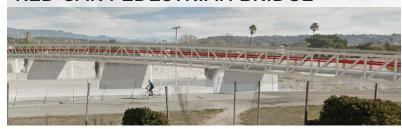
The **Red Car Pedestrian Bridge** is a footbridge built on the supports once used for the Red Car Trolley.
