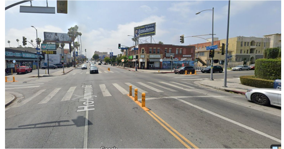
Left turn calming at Hollywood Bl and Normandie Ave
