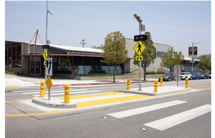
Pedestrian flashing beacon and concrete refuge island at Hollywood/Rodney
