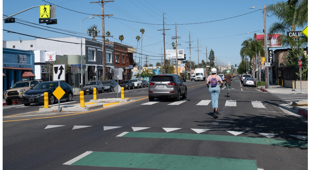
Similar lane reconfiguration with conventional bike lane on Adams Blvd in West Adams
