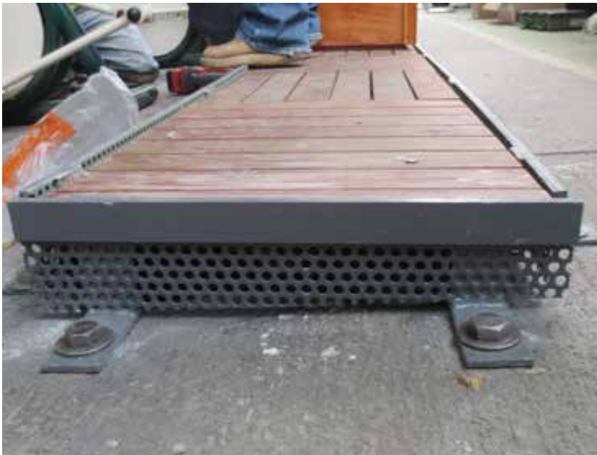
Perforated-steel Parklet perimeter allows for proper drainage of stormwater
