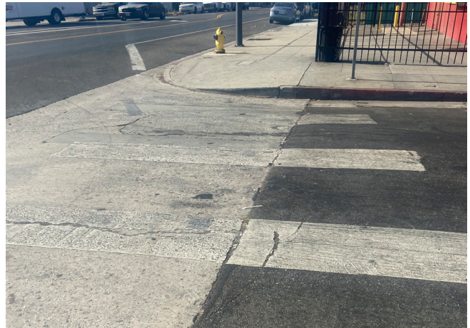
Crosswalk with faded striping
