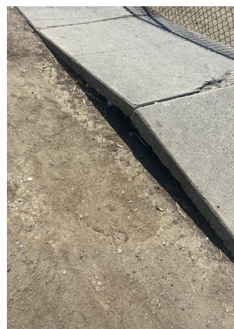
Cracked sidewalks on Imperial Highway
